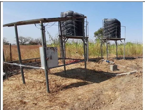
The solar panel, Bhungroo and overhead tanks in Sepaat field (Picture: Henry E. Igbadun)
