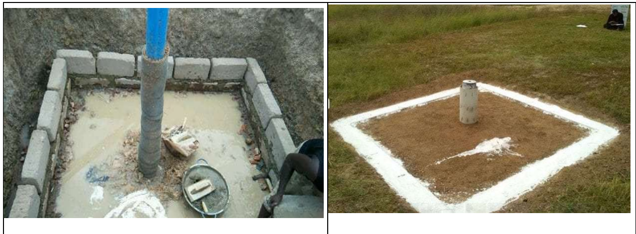
Figure 4: Typical filtration system of the Bhungroo (source: Engineering for Change, 2022):
